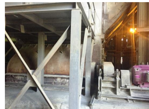
Mills and Crushers
