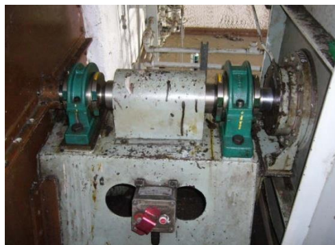
Fans and Blowers
